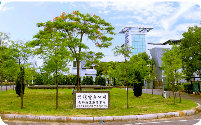
STSP Extra High Voltage Substation
