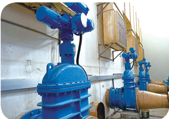
Upgrade and Replacement of Water Control Valves
