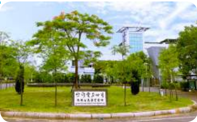
STSP Extra High Voltage Substation
