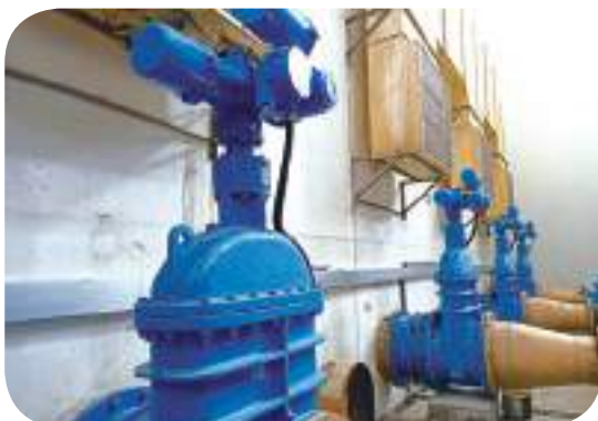
Upgrade and Replacement of Water Control Valves
