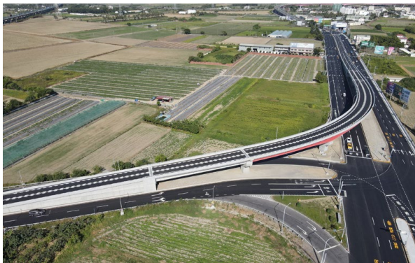
Photos of Xingangshe Boulevard diversion project site
