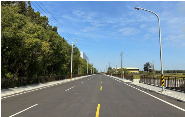
Photos of the South 137 widening project site
