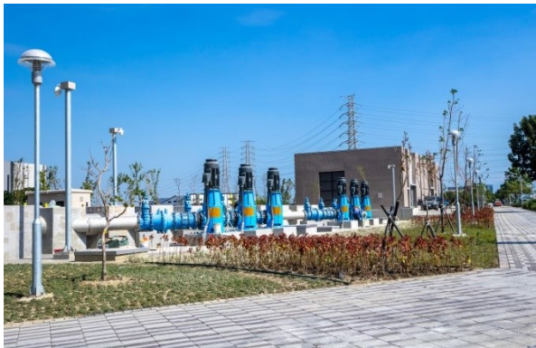
Photos of the completed sixth distribution reservoir in Tainan Science Park
