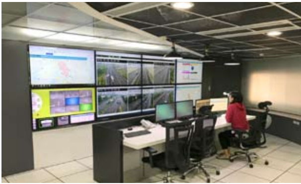
▲ The STSP Traffic Control Center (2018/2/9)
