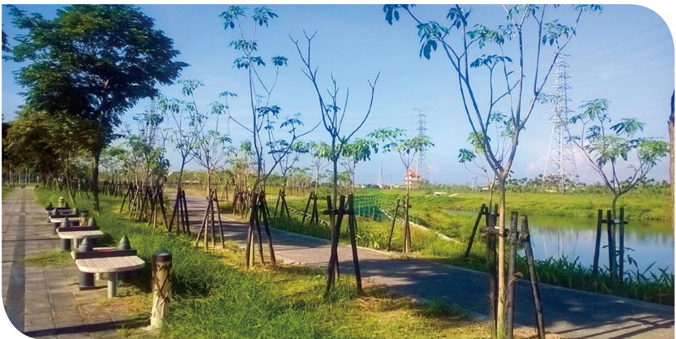
■ Finishing work on detention basin A at the KSP (06/06/2016)
