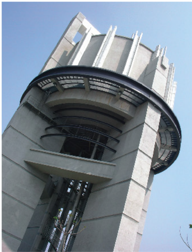
> The Second Elevated Tank
