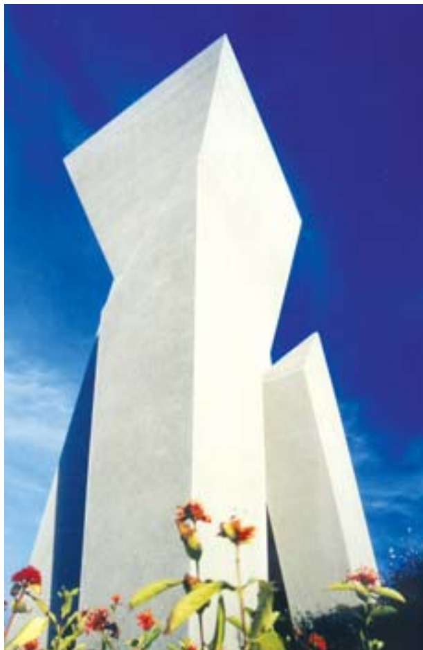
Figure 2-4 General Water Tank of Tainan Science Park
