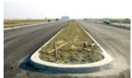
Figure 5-6-12 Lujhu Science Park's Phase 1 Zone 1 Road Construction Project
