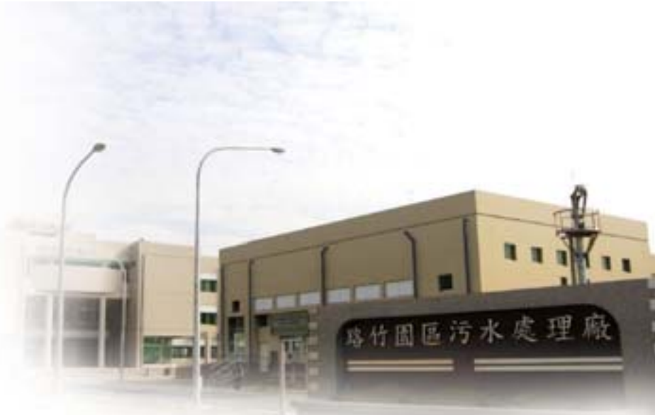
Figure 5-6-8 Lujhu Science Park's Waste Water Treatment Plant - Phase 1
