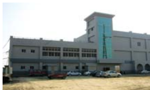
Figure 5-6-14 Taiwan Power Company's Extra High Voltage Substation at Lujhu Science Park ( to be completed in June 2004 )
