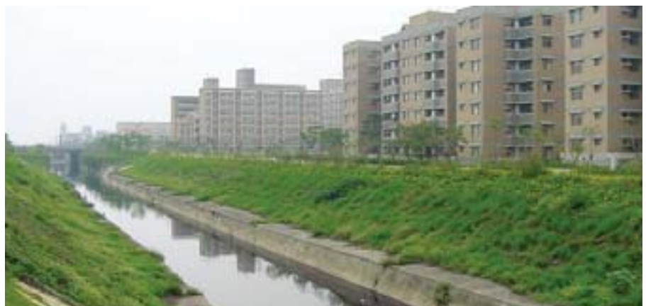
Figure 5-5-3 Flood-prevention Drainage Project Completed
