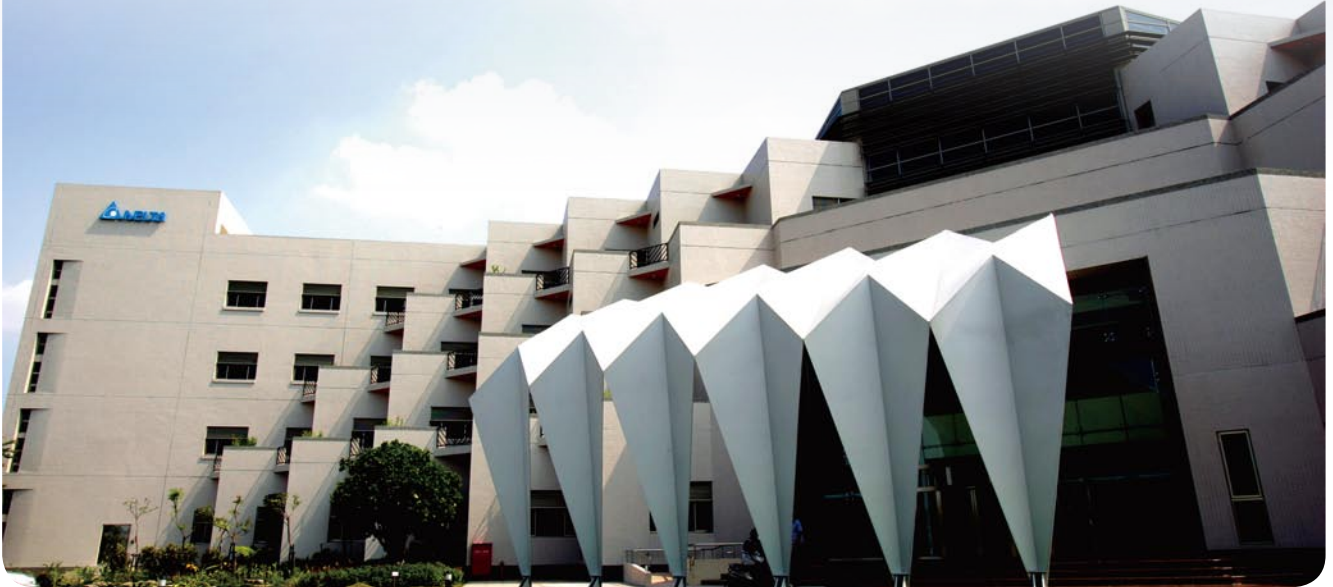
■ The Green Factory at the TSP — Phase I Factory of Delta
