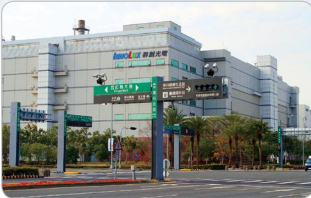
■ Recognizable and Systemized Road Guidance System at the STSP
