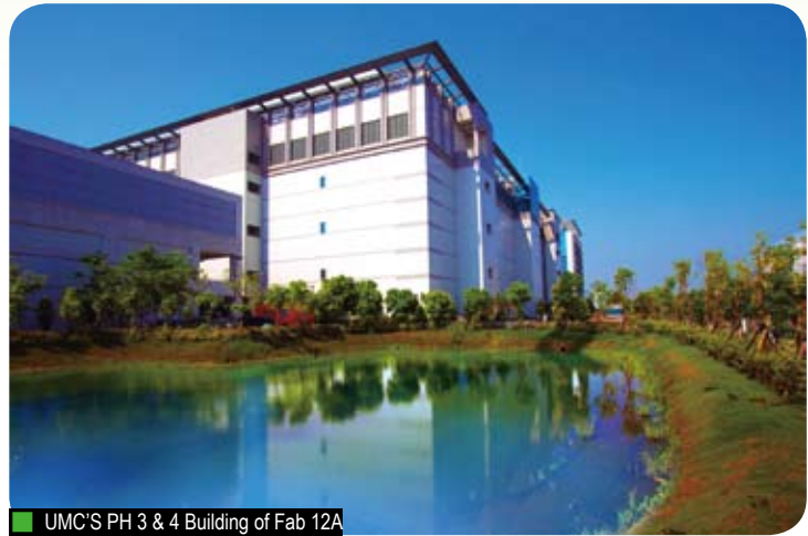
■ UMC'S PH 3 & 4 Building of Fab 12A
