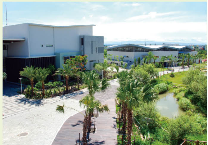
▼ "Diamond Level Green Building Labeling" Building at the NNKIEH
