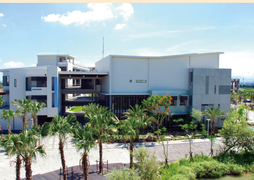
▼ NNKIEH is the first school obtained the Diamond Level Green Building Labeling in Taiwan
