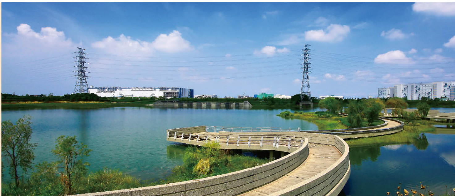
▼ Flood Prevention Function of the Detention Ponds at the STSP
