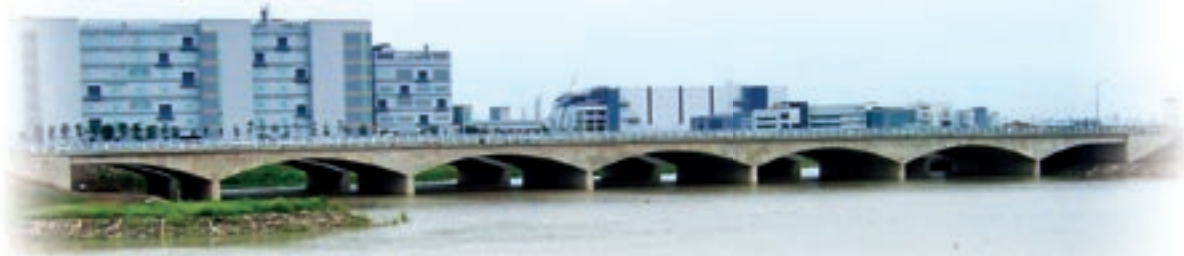
Tainan Science Park Northwest Region, Sub-Region II Site, Nanke 9th Rd. variable-depth box girder bridge complete
