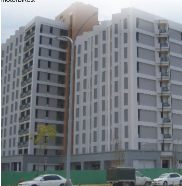
The First-phase Employee Dormitory in the KSP
