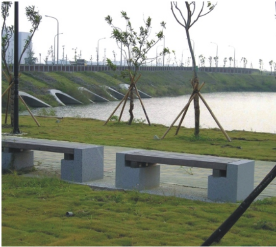
Newly Built Five-hold Culverts Constructed beneath the 40-meter Roadway to Connect the Detention Ponds on the Northern and the Southern Sides
